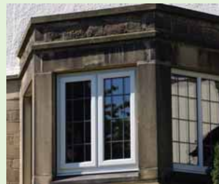
Original dressed stone bay window with replacement leaded glass
