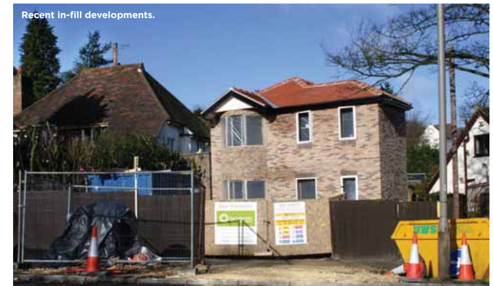
An original bungalow and side garden replaced by two detached houses in 2010.
